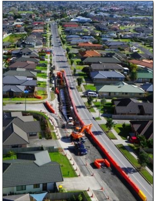
Figure 6: example of construction area with traffic management
