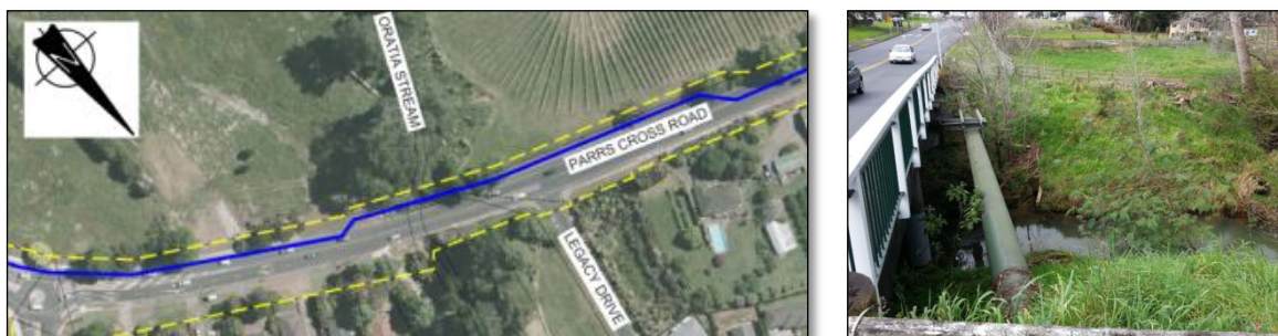
Figure 20: Existing Oratia Stream with pipe and road crossing
